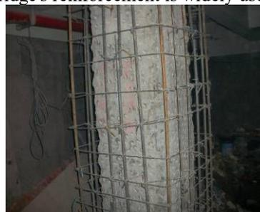
Figure 4. Increasing section reinforcement method
