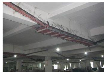
Figure 3. External prestressing reinforcement method
