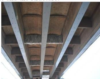
Figure 2. Bonded steel plate reinforcement method
