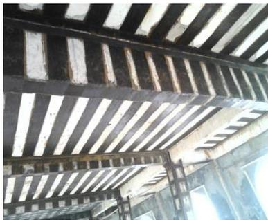
Figure 1. Bonded carbon fiber reinforcement method
