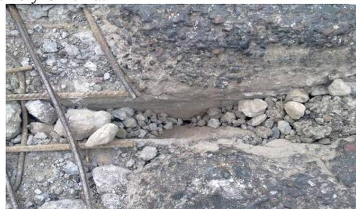
FIGURE 2. The destruction of hinge seam
